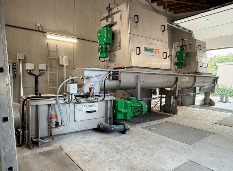
An installation by Envirosep featuring 2 STRATOSEP screens, 1 ENVIROSPIR screw conveyor and 1 SPIRAPRESS screw washer-compactor.
